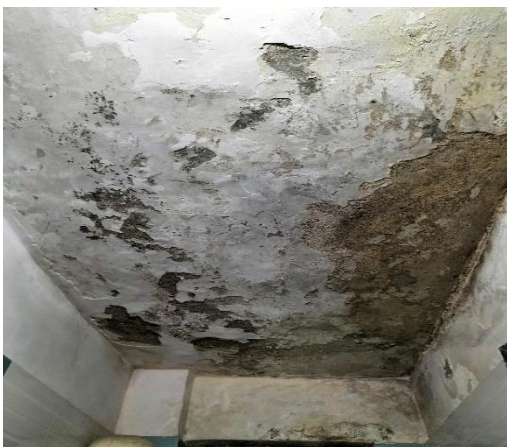
Leakages in Slab
