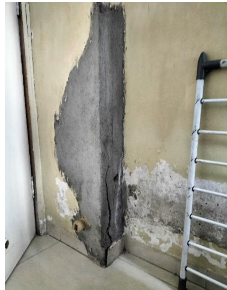
Cracks in repaired Column
