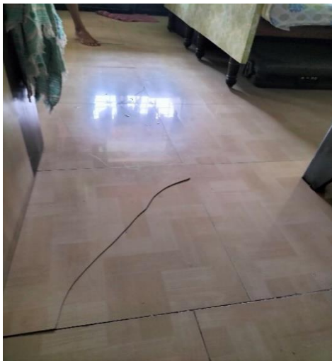
Cracks in Flooring
