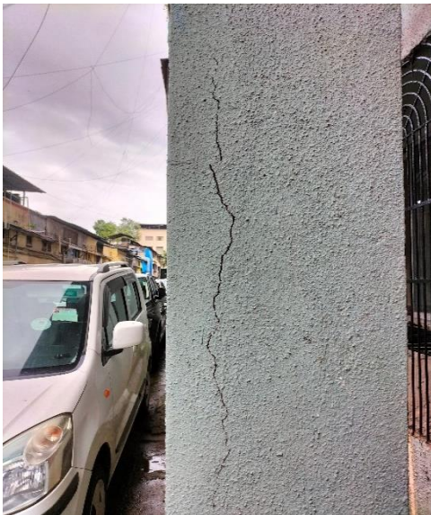
Cracks in repaired Column
