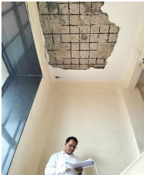
Collapse of Slab
