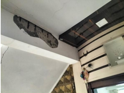
Cracks in Beam and Slab
