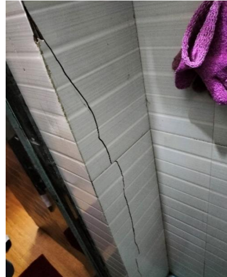
Cracks in Column
