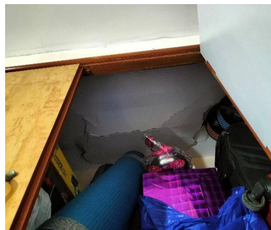
Cracks in Slab
