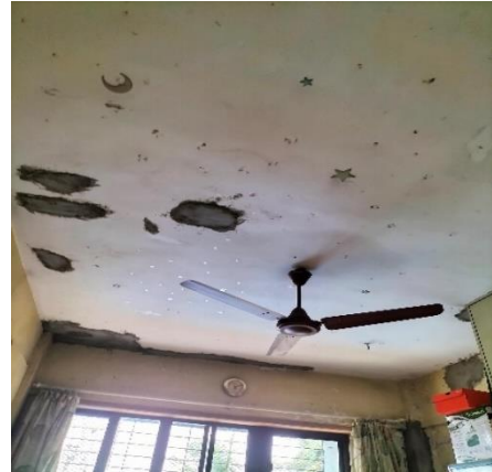
Cracks in Beam and Slab
